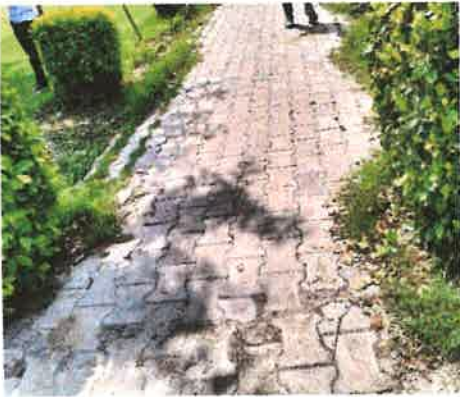
Paving stone installed in campus
