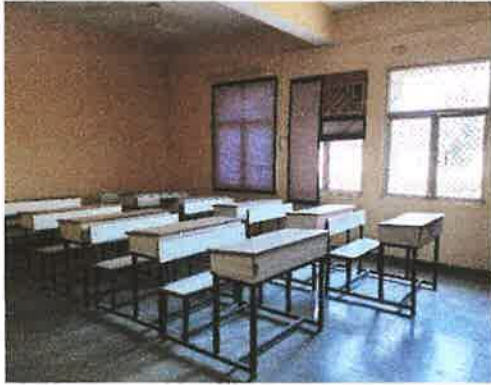
Classrooms as per NBC guidelines with more than 40% window ratio
