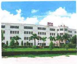
Well ventilated building structure
